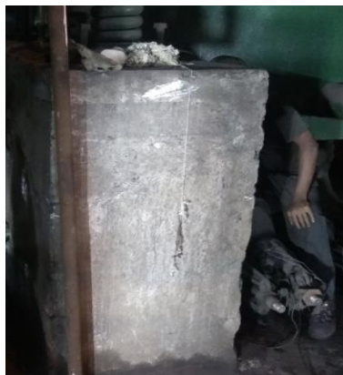
Pedestal Structure where opposite faces are accessible (Direct)
