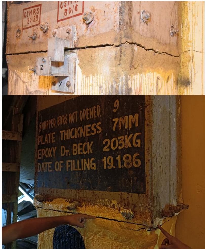
Cracks Observed in the Penstock Gallery Columns
