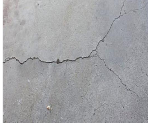
Appearance of Surface Cracks in Concrete
