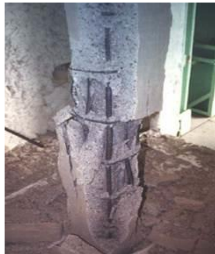
Fire effects on Concrete column
