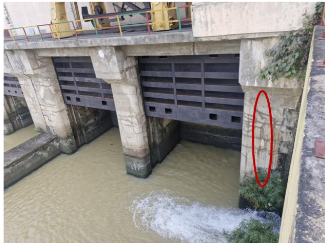
Damages in Wall, Piers, Breast and Divide Walls of Rihand Dam, UP
