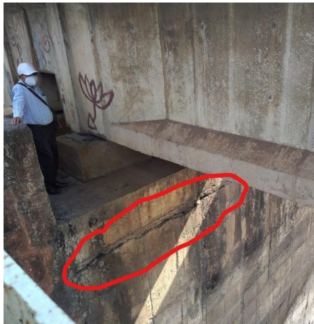
Cracks Observed in Pier
