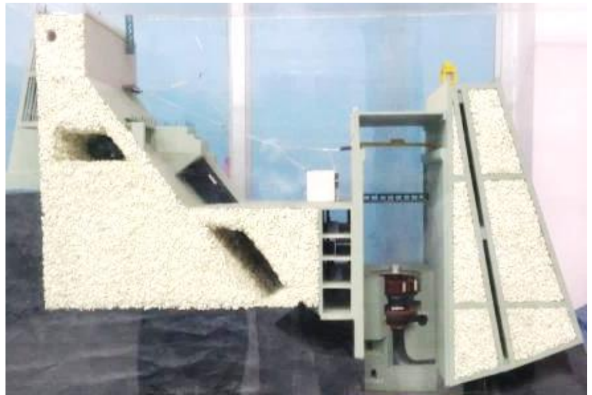
Cross sectional model of Kadana Dam Power House (Photo courtesy: Kadana Dam Authority)
