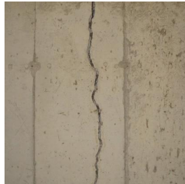
Appearance of Cracks in Concrete due to Settlement
