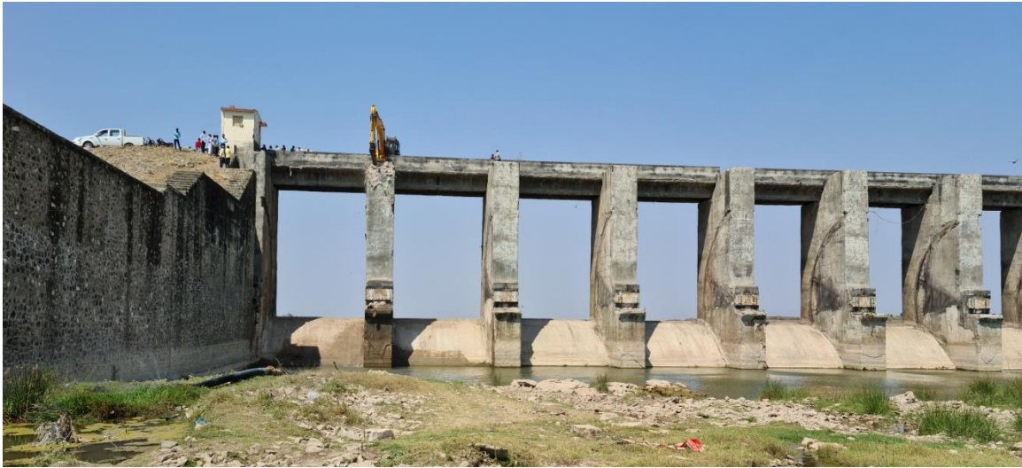
Dismantling of Old Spillway in Progress
